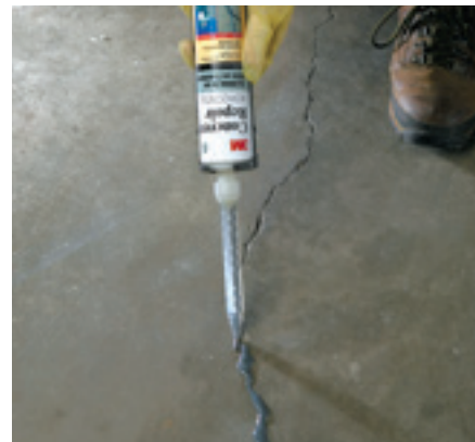
Self-leveling concrete repair: 3M™ Concrete Repair 600 ( pg 26 )
